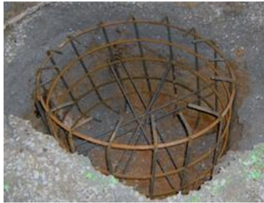
Figure 17: Footing Reinforcement
