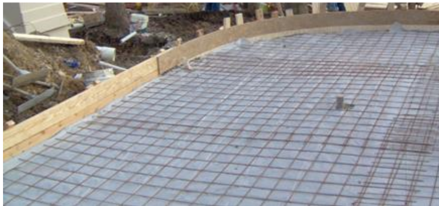
Figure 30: Moisture Barrier on Pad
