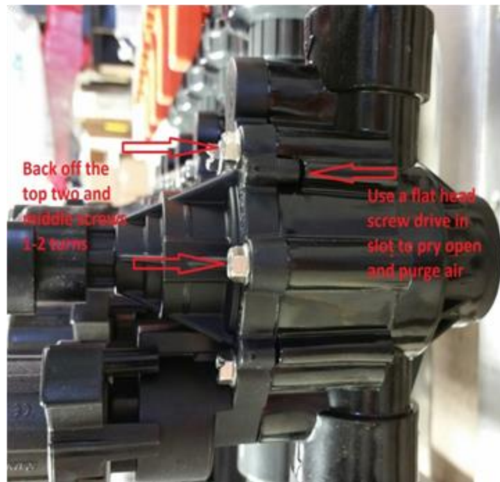
Figure 7: Water Hammer Procedure
