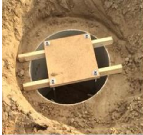
Figure 18: Footing Template & Anchor Bolts
