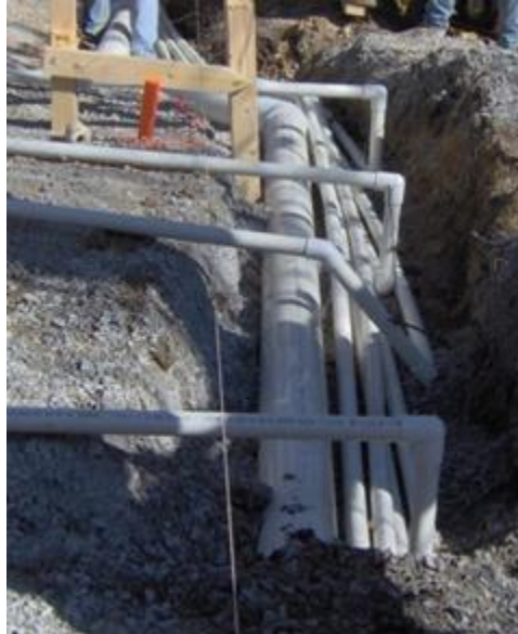
Figure 23: Drain Lines for a Spray Park
