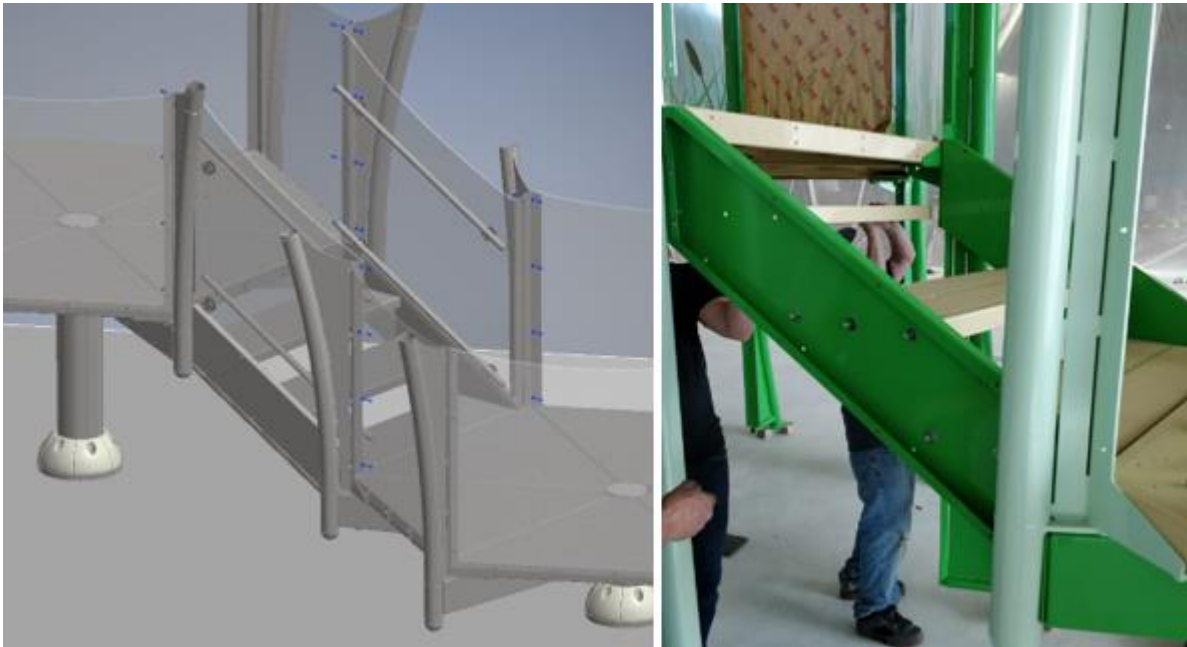
Figure 17: Transition Stairs Assembly
