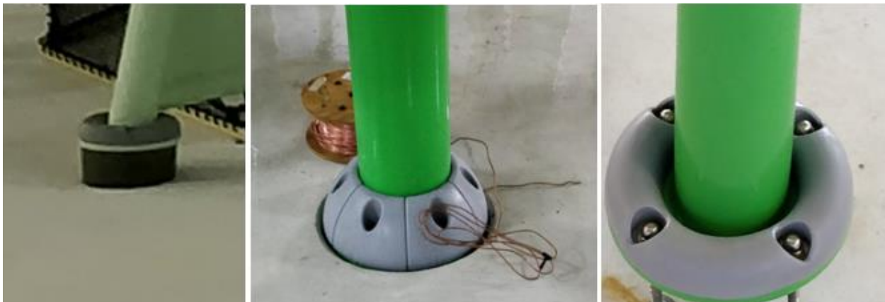
Figure 9: Installed Main & Support Columns
