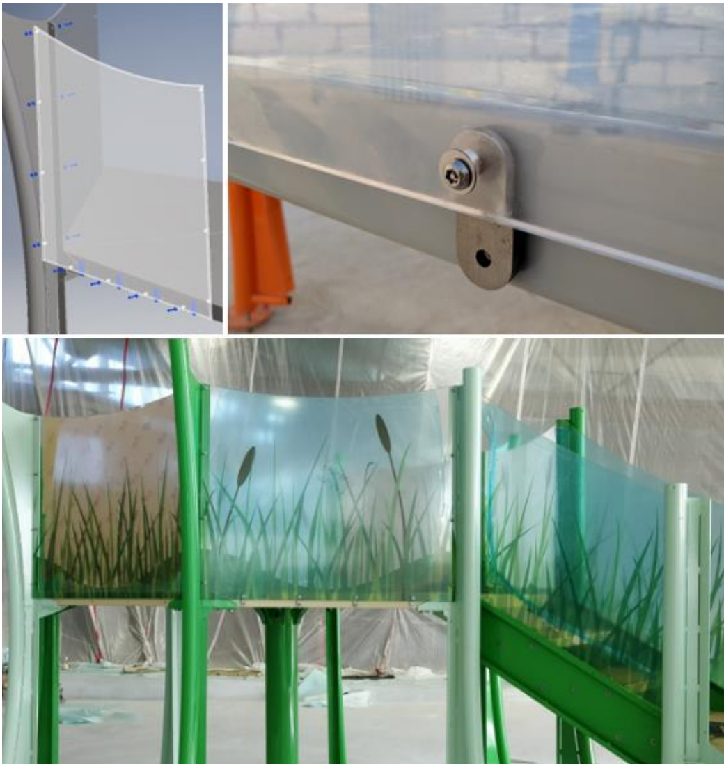
Figure 18: Panel Installation
