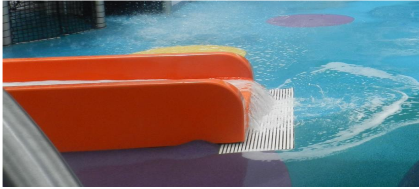
Figure 20: Flume Run Out
