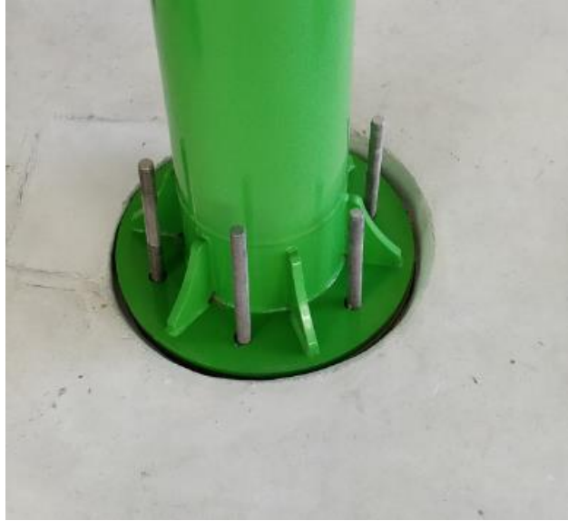
Figure 2: Baseplate with Pad Leveling
