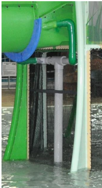
Figure 19: Flume Installation & Plumbing
