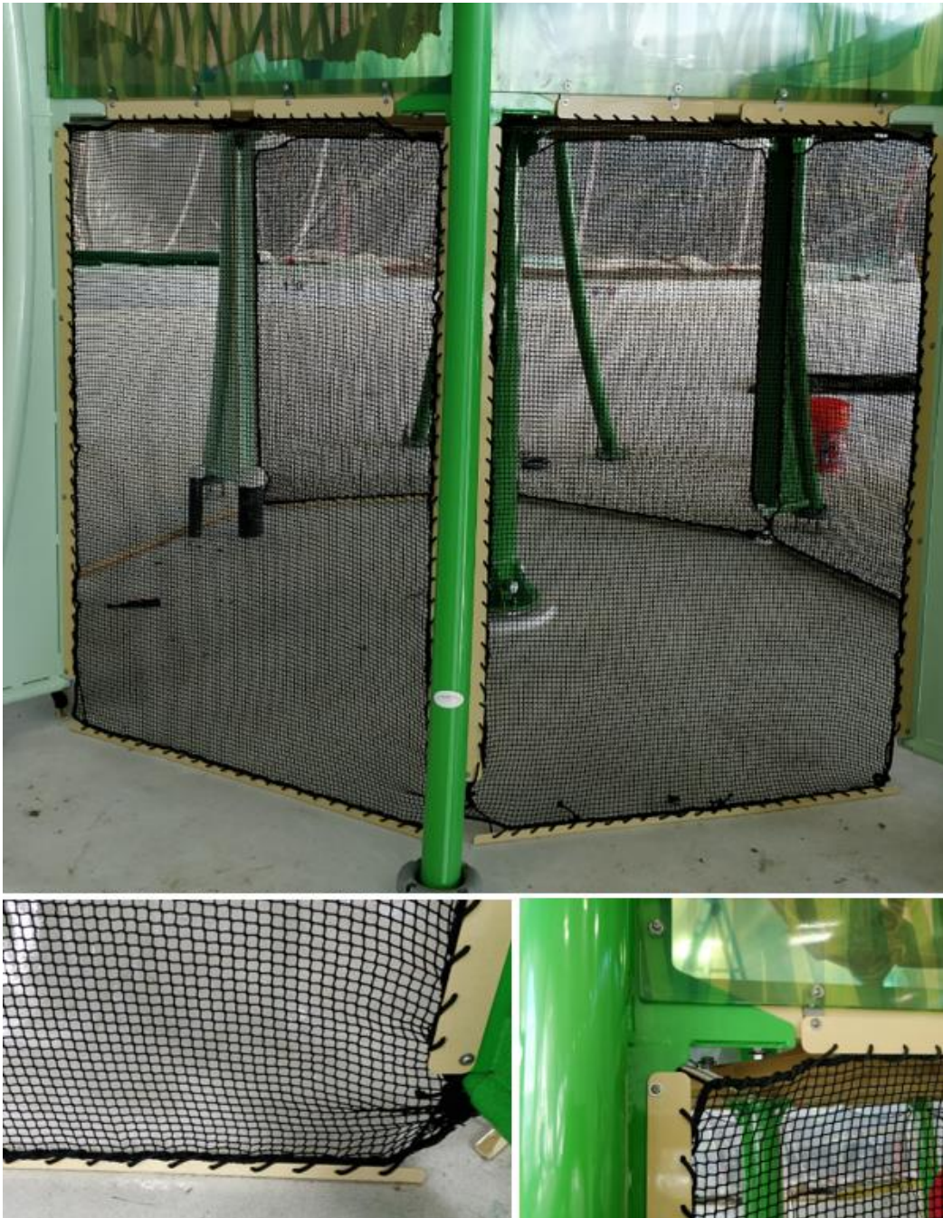
Figure 31: Play Pod Octo Netting Installation
