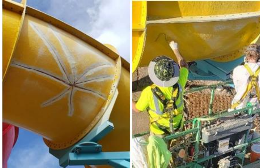
Figure 63: FRP Deformation Repair Grinding and Fiberglass Application
