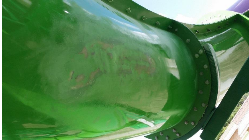
Figure 45: Sanded and Cleaned Putty on Fiberglass Repair, Outside
