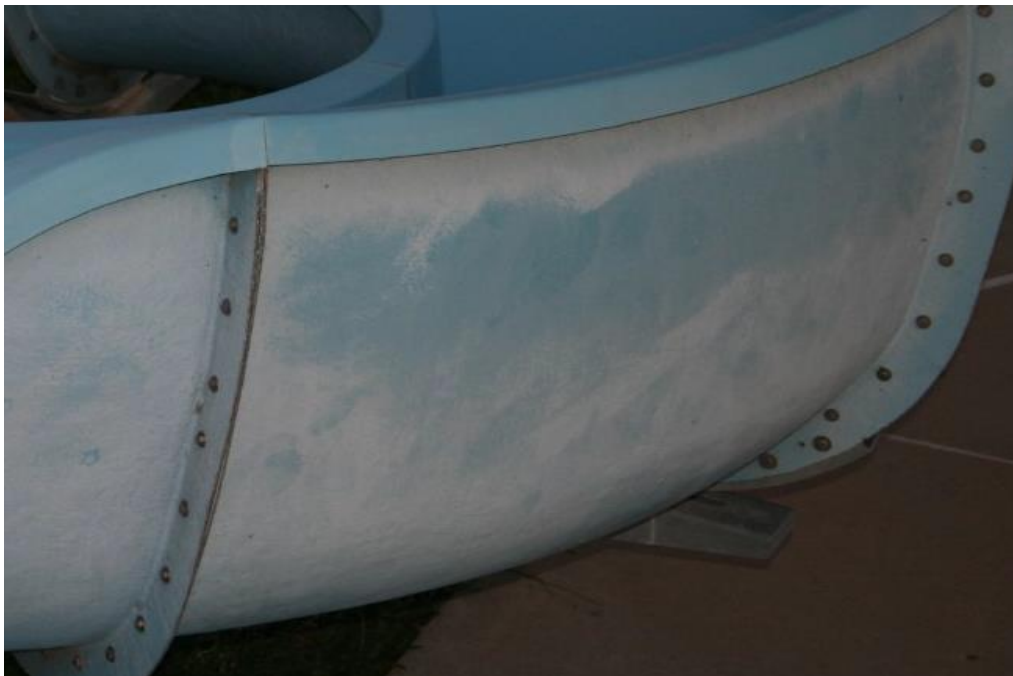
Figure 24: Faded Clear Coat DC92
