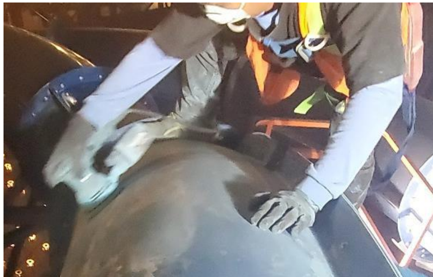
Figure 70: Sanding FRP for Clear Coat
