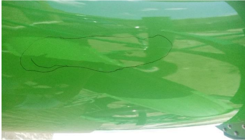
Figure 27: Marked Area for Repairs
