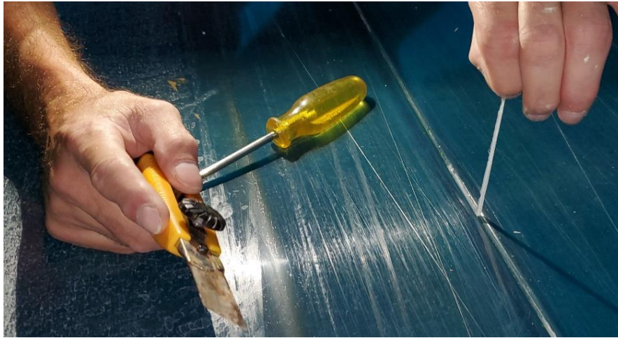
Figure 7: Removing Old Filler
