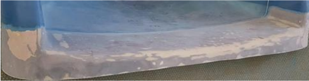
Figure 60: Sanded Gelcoat Ready for Barrier Coat
