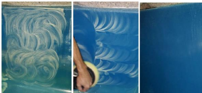
Figure 6: Buffing and Waxing Shutdown Lane FRP
