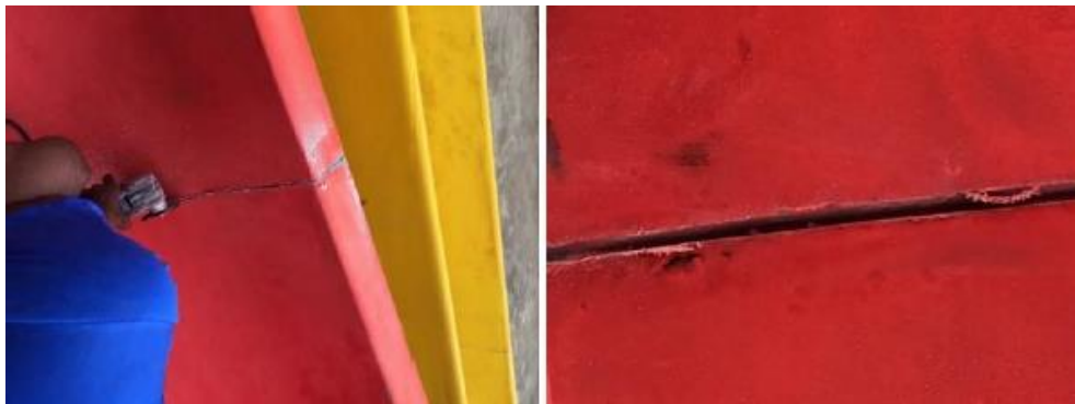
Figure 8: Mechanically Remove Filler and Deburr Edges
