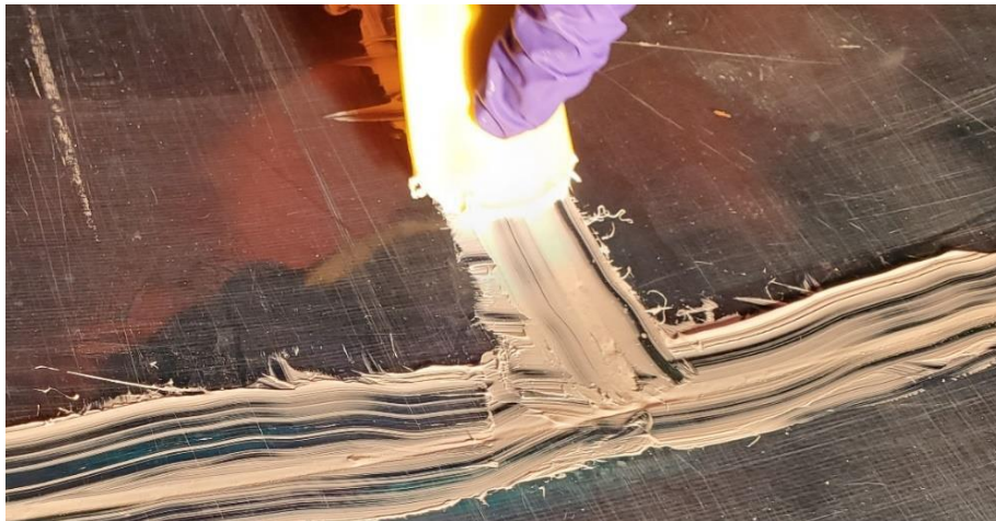
Figure 12: Press in New Filler
