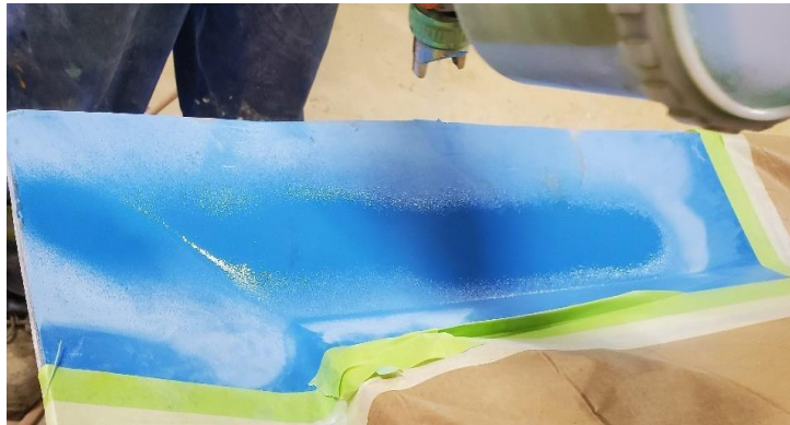
Figure 53: Spray on an Even Coat
