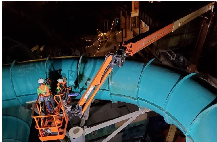
Figure 69: Use Proper Height Access and Fall Protection Equipment
