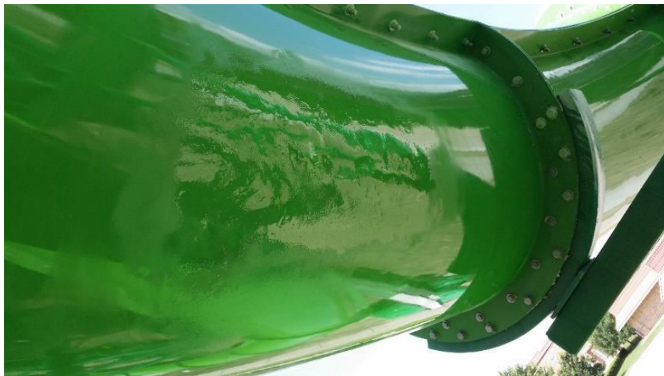
Figure 56: Gelcoated Large Repair, Outside
