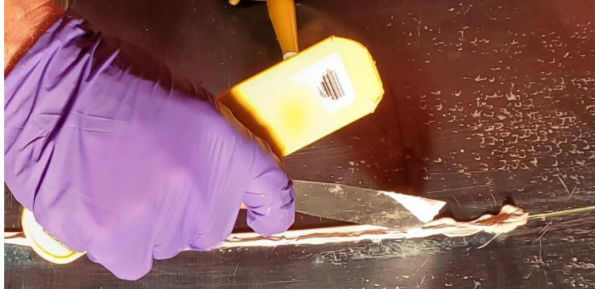
Figure 11: Pack in Joint Filler
