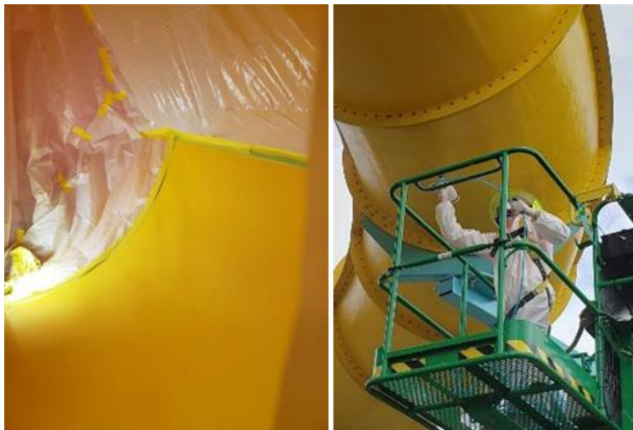
Figure 64: FRP Deformation Repair Gelcoat and Clear Coat Finishing
