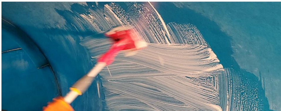
Figure 5: Scrubbing Calcium, Lime, and Rust Remover on FRP
