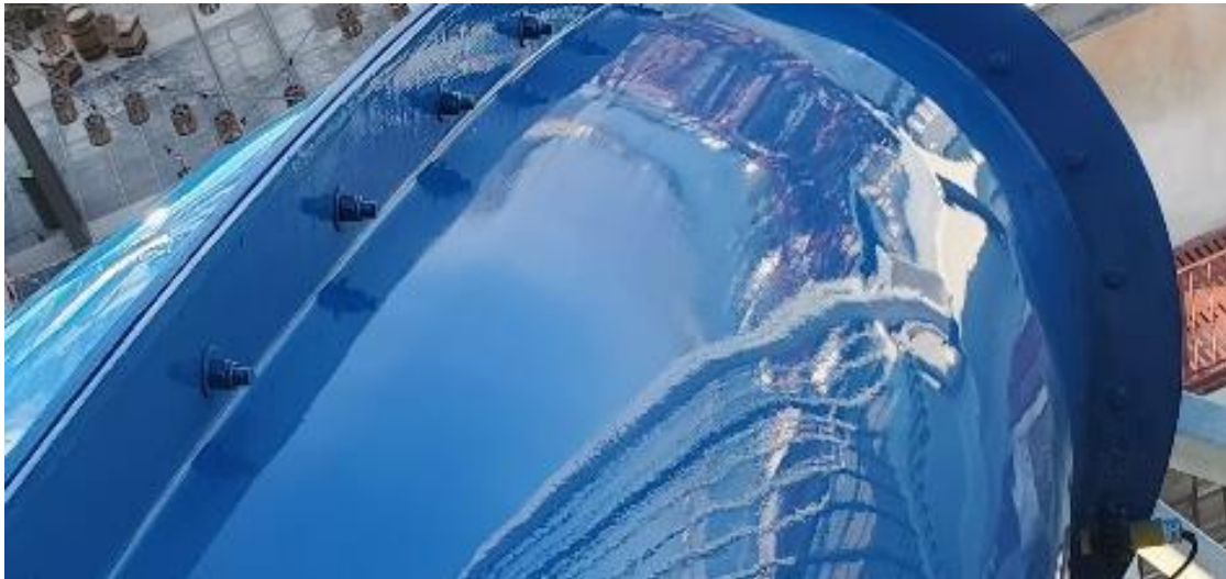
Figure 73: Inspect Finished FRP for Drips or Runs
