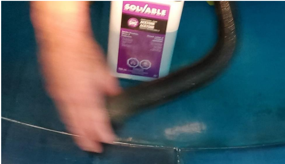
Figure 9: Vacuum and Clean Joints with Acetone
