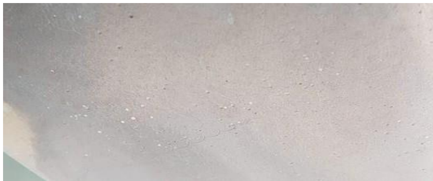
Figure 61: Pinholes in FRP Need Filling before Barrier Coat
