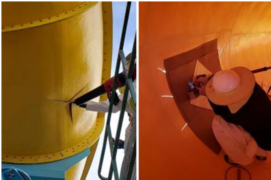
Figure 62: FRP Deformation Repair Preparation
